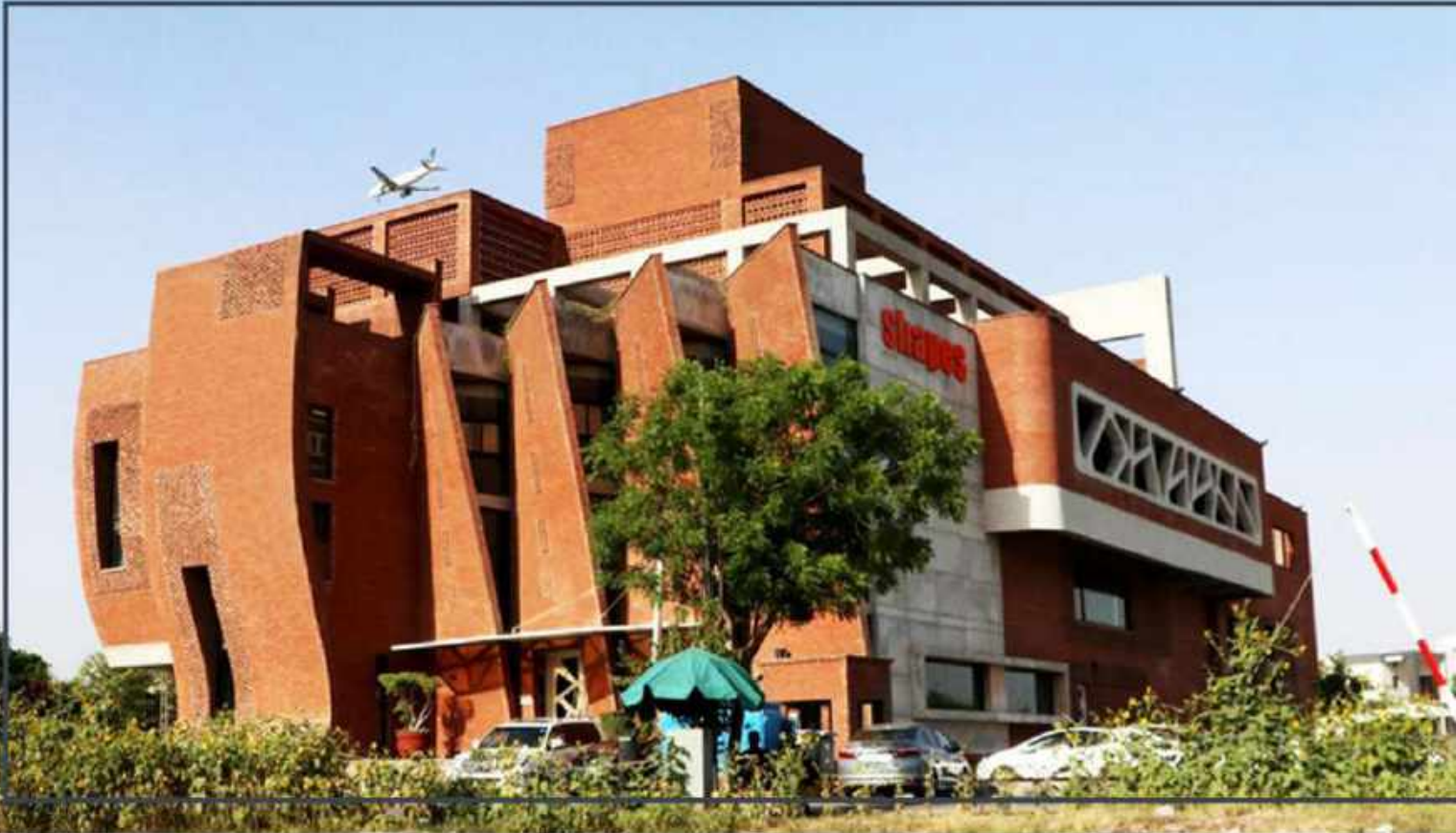
Structural & Interior works of Shapes Club DHA, Lhr.-2012
